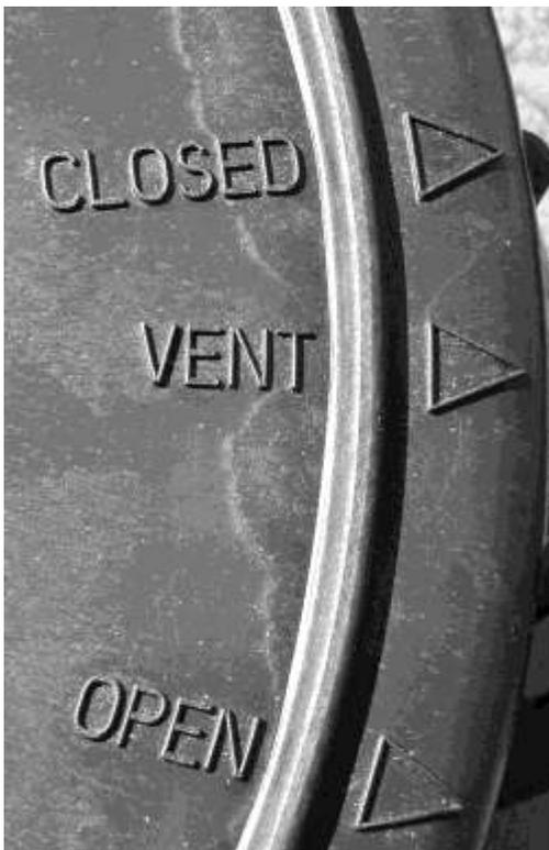
Place the lid on the unit by using the aligning arrows. Notice there is three (3) settings marked on the lid **OPEN**, **VENT**, and **CLOSED** with an aligning arrow to the right of each (shown on left here).
